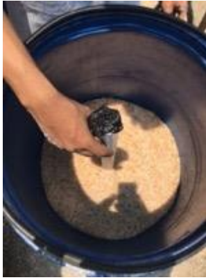
Gambar 12 Penataan Media Filter Air
